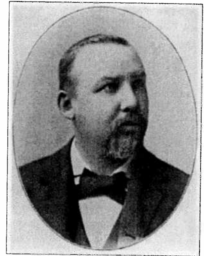
The Heyworth Building was built by Otto Young, a wholesale jeweler and real estate investor involved in the development of State Street and Wabash Avenue as premier shopping streets in Chicago.
